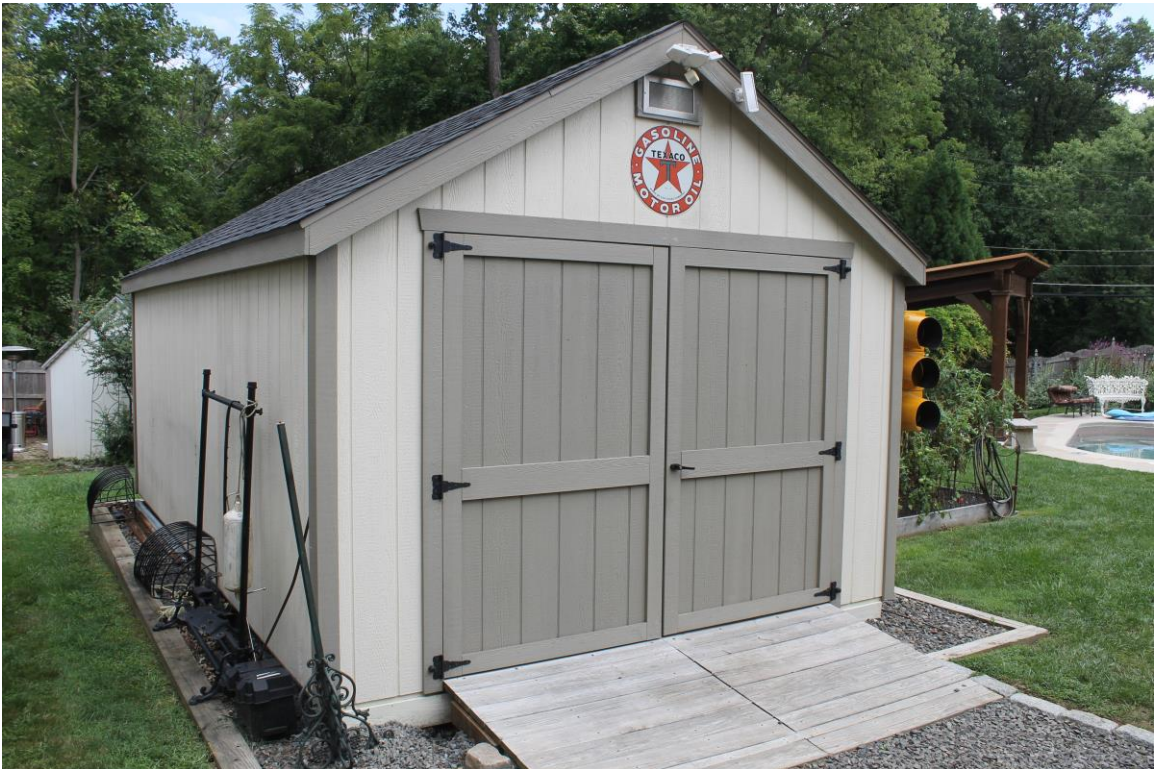
Photograph 10: The northwest (side) and southwest (front) elevations of the modern shed, camera facing east (August 2024).
