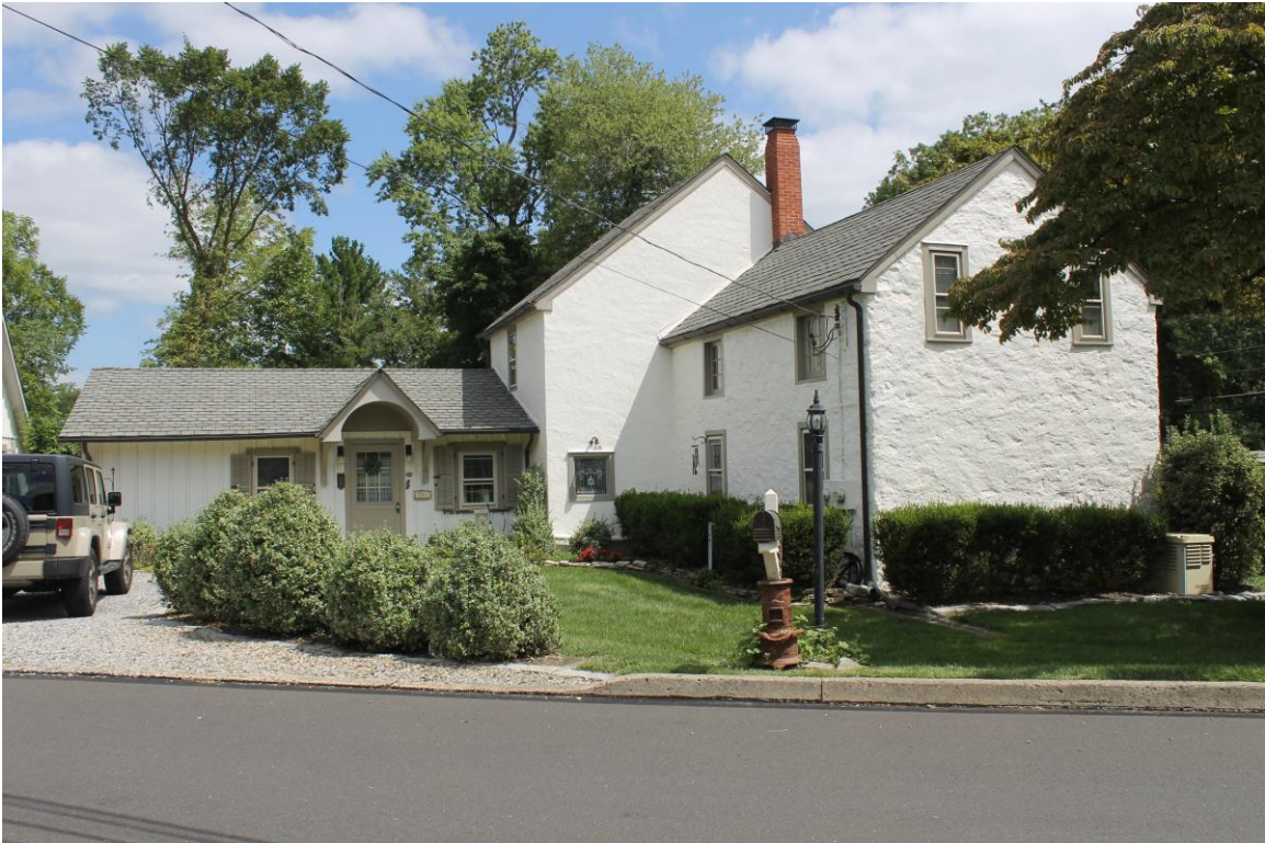
Photograph 2: The southwest (side) elevation of the dwelling, camera facing northeast. Note the one-story addition and converted garage (left), the pre-1938 two-and-a-half-story addition (back middle), and the pre-1890 two-story main block of the dwelling (front right) shown here (August 2024).
