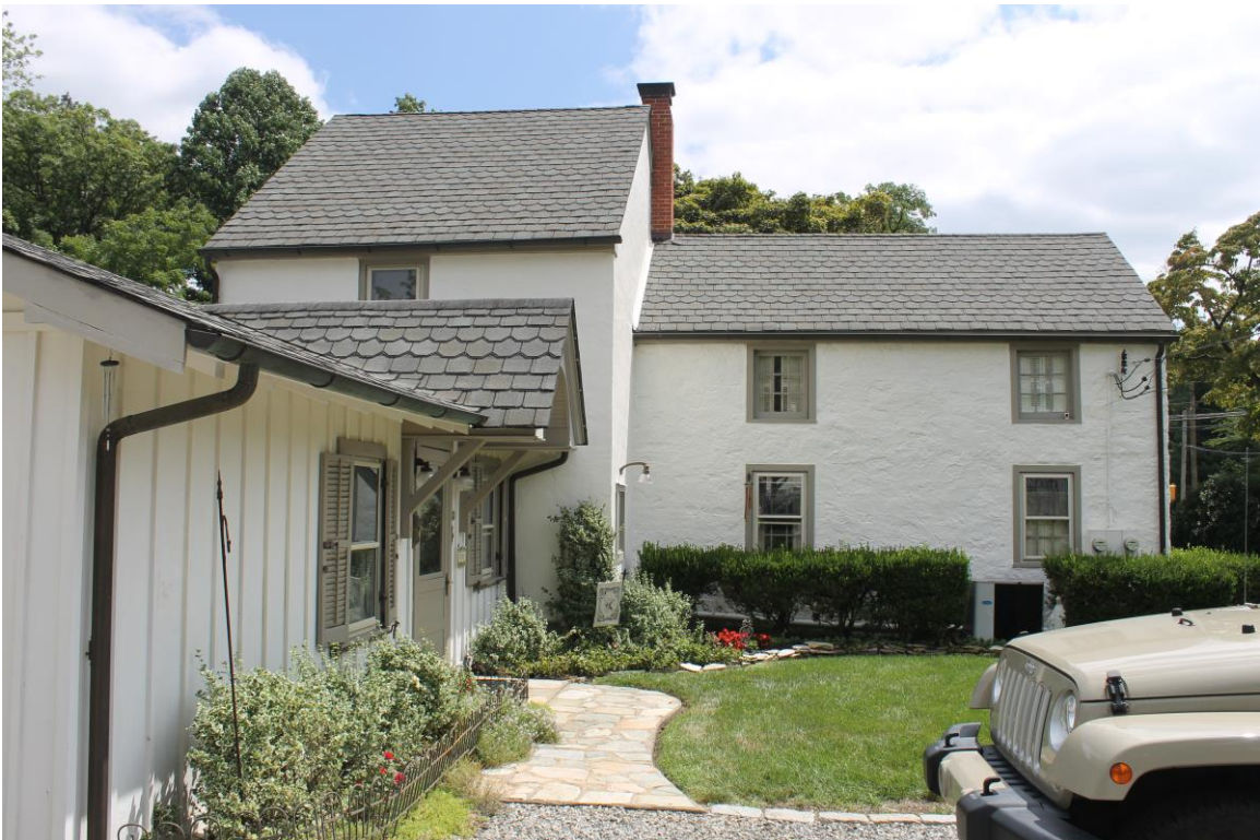
Photograph 4: The northwest (rear) of the dwelling showing the one-story addition and converted garage (front left), the pre-1938 two-and-a-half-story addition (back center), and the pre-1890 two-story main block of the dwelling (right) (August 2024).
