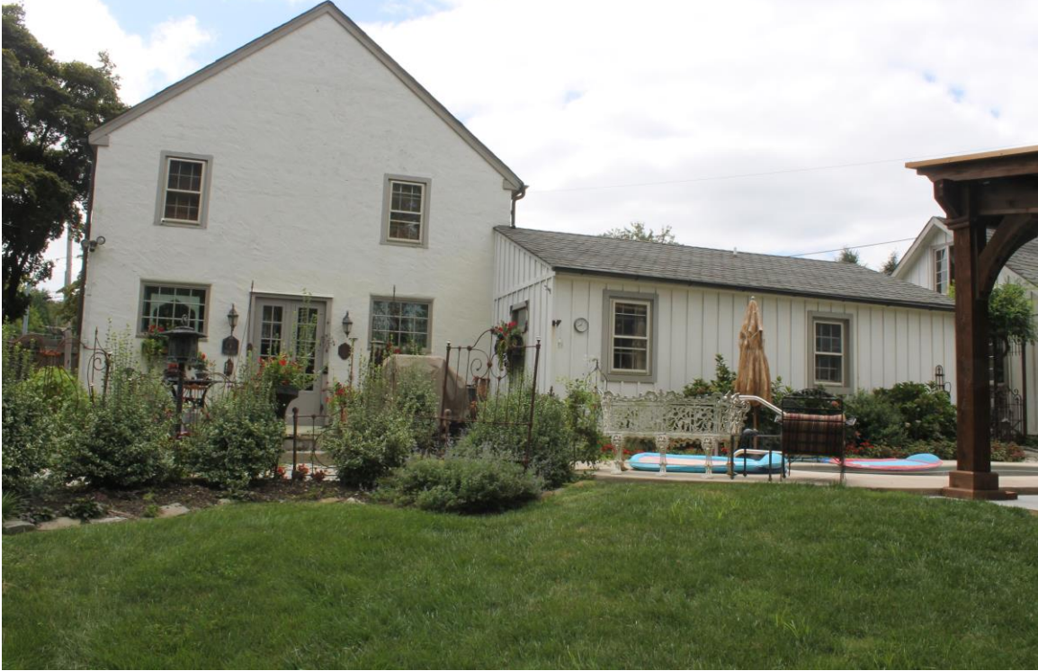
Photograph 5: The northeast (side) of the dwelling showing the pre-1938 two-and-a-half-story addition (left) and the one-story addition and converted garage (right), camera facing southwest (August 2024).
