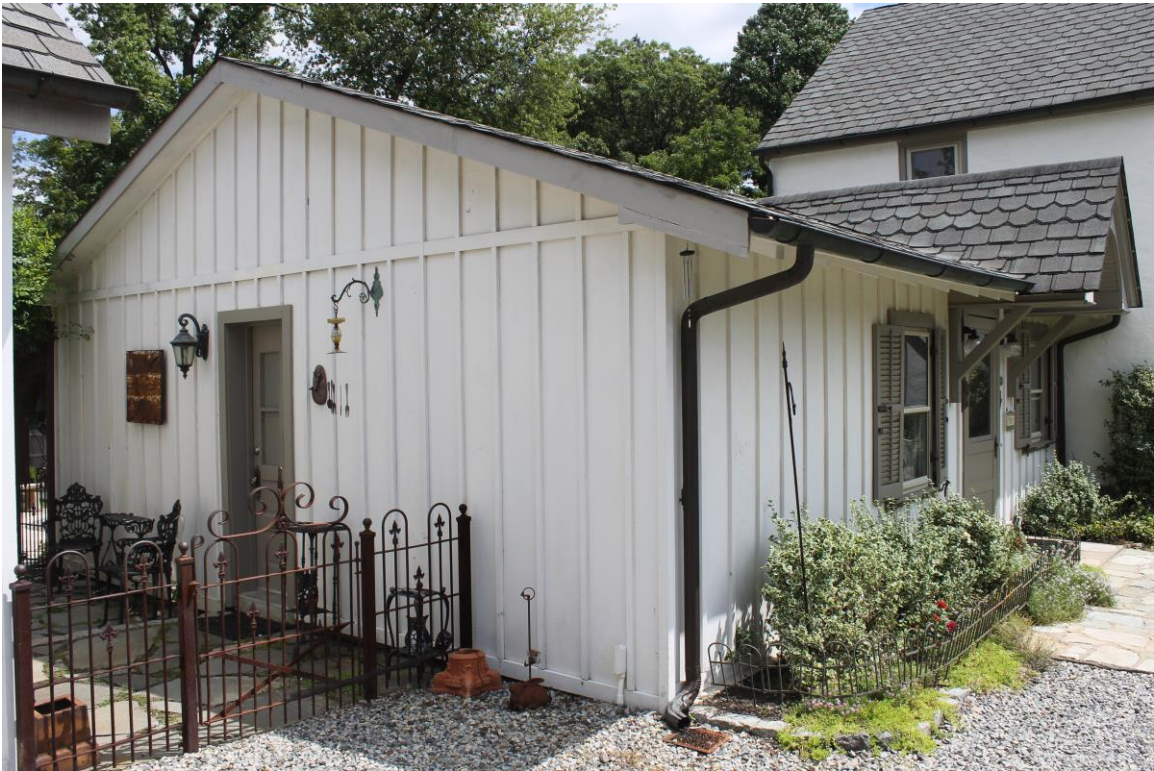
Photograph 3: The northwest (rear) elevation of the dwelling, camera facing east. Note the one-story addition and converted garage (front left) and the pre-1938 two-and-a-half-story addition (back right) shown here (August 2023).
