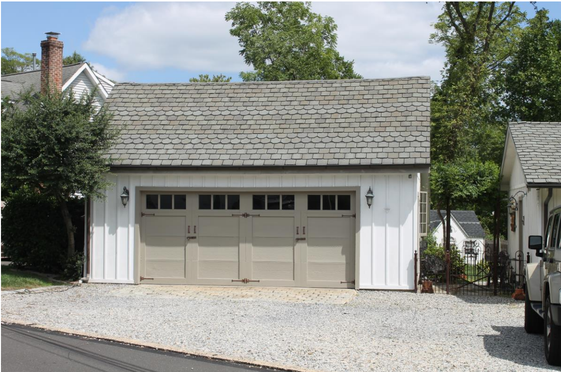
Photograph 6: The southwest (primary) elevation of the 2003 garage, camera facing northeast (August 2024).
