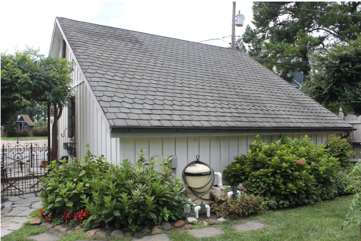
Photograph 8: The northeast (rear) elevation of the 2003 garage, camera facing west (August 2024).
