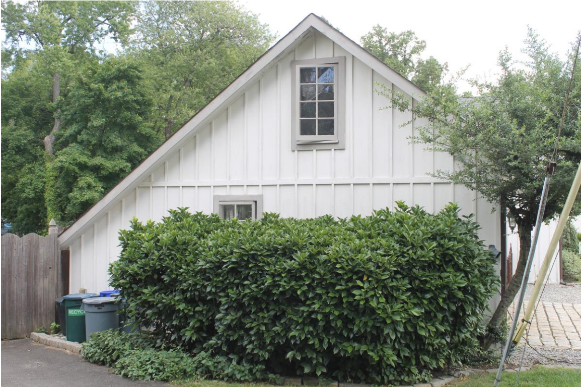
Photograph 7: The northwest (side) elevation of the 2003 garage, camera facing southeast (August 2024).
