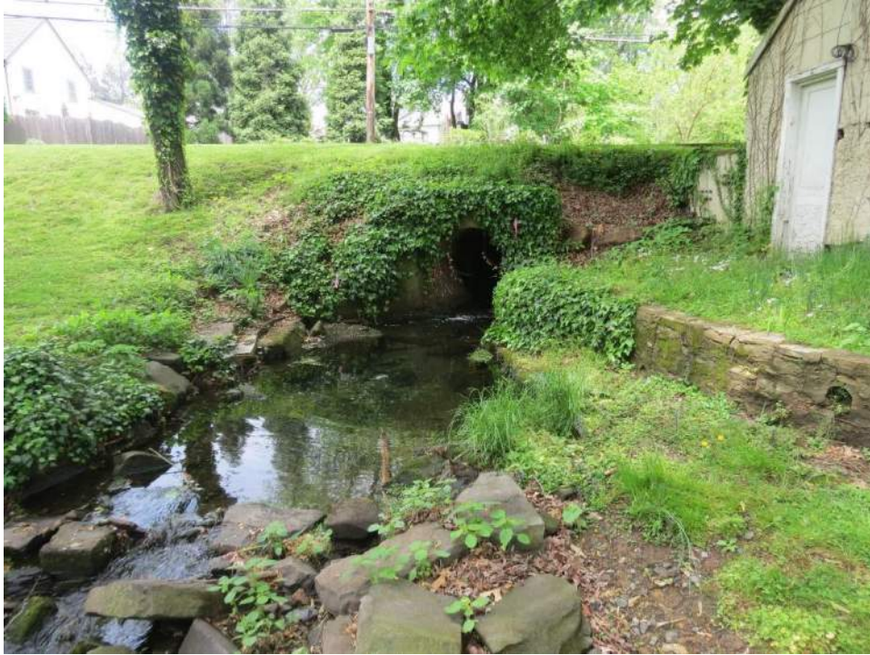
Photo 25: Looking northwest (upstream) along WUS-6, towards the culvert crossing beneath SR 2045 (Old Lincoln Highway). Photo taken May 4, 2021.
