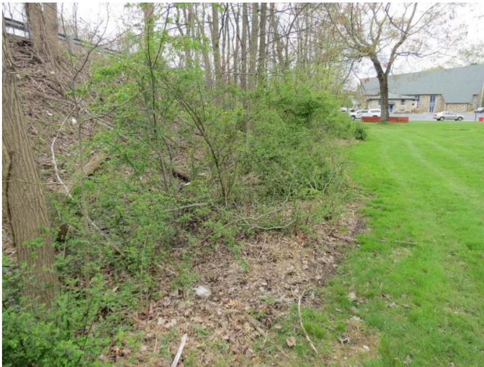
Photo 8: Looking southwest along the toe of slope on the north side of the West Gillam Avenue roadway embankment, to the west of SR 0413 (S. Pine Street). Photo taken April 19, 2021.
