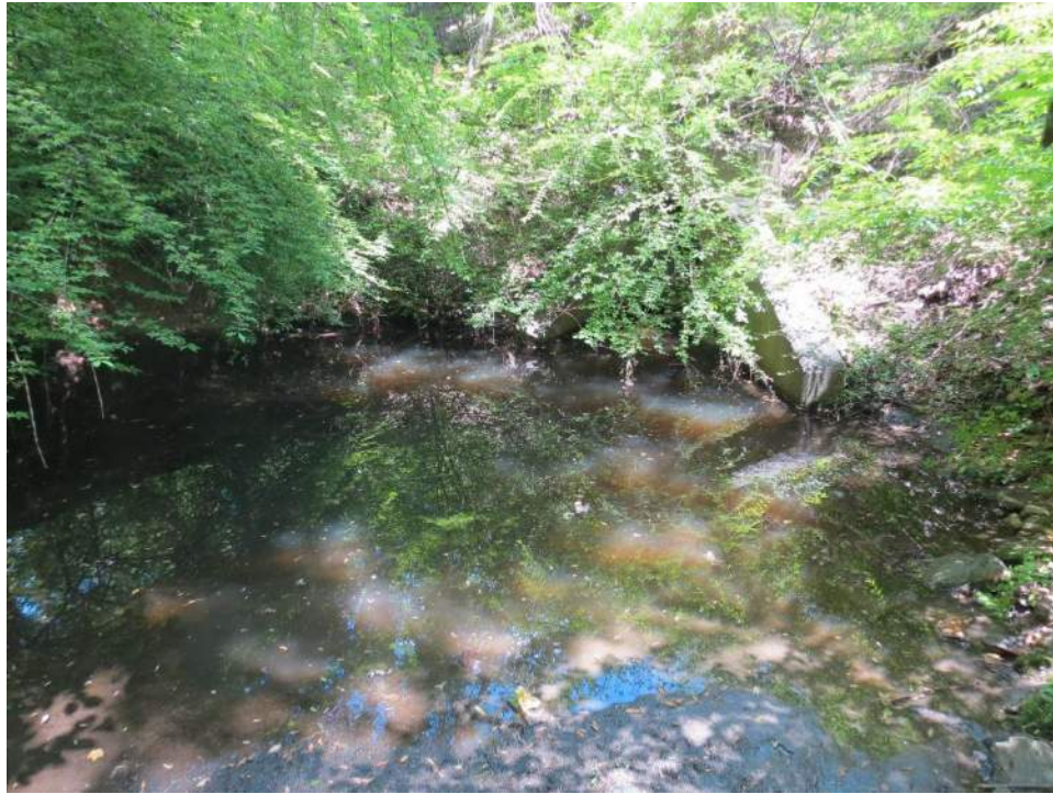
Photo 63: Looking northeast (upstream) along WUS-14, towards the culvert crossing beneath West Interchange Road. Photo taken May 11, 2021.
