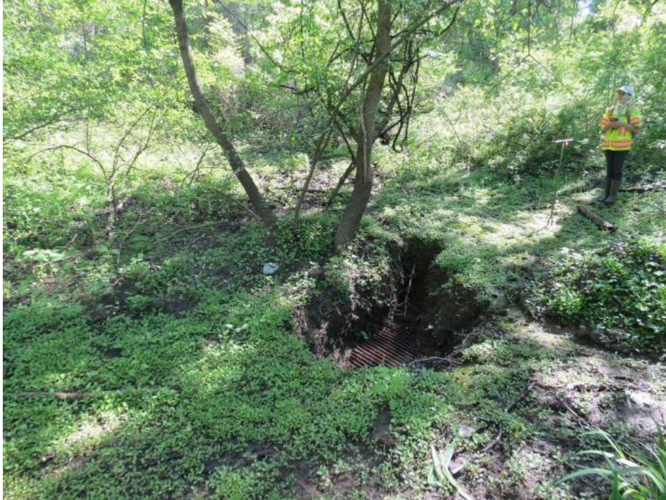
Photo 52: Looking northeast towards a constructed stormwater inlet located between SR 2008 (Highland Avenue) and Park Avenue, to the south of SR 0001. Photo taken May 11, 2021.
