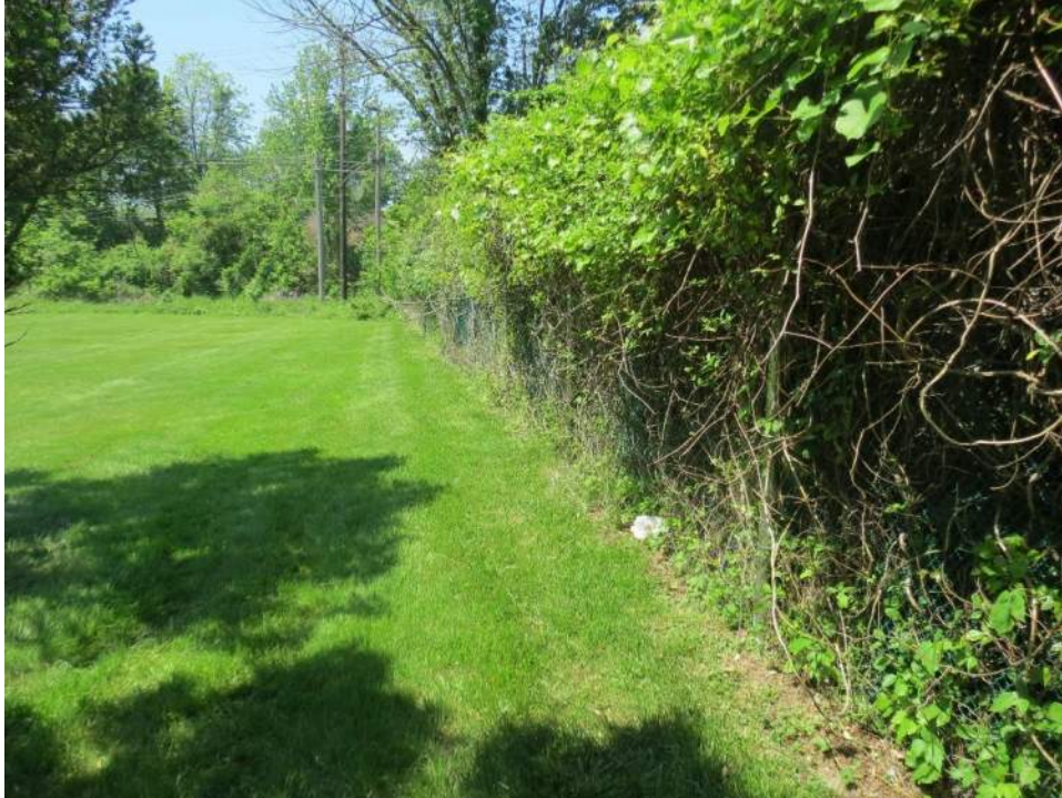
Photo 76: Looking southwest along the roadway ROW fence located south of SR 0001 and east of SR 0413 (Pine Street). Photo taken May 19, 2021.
