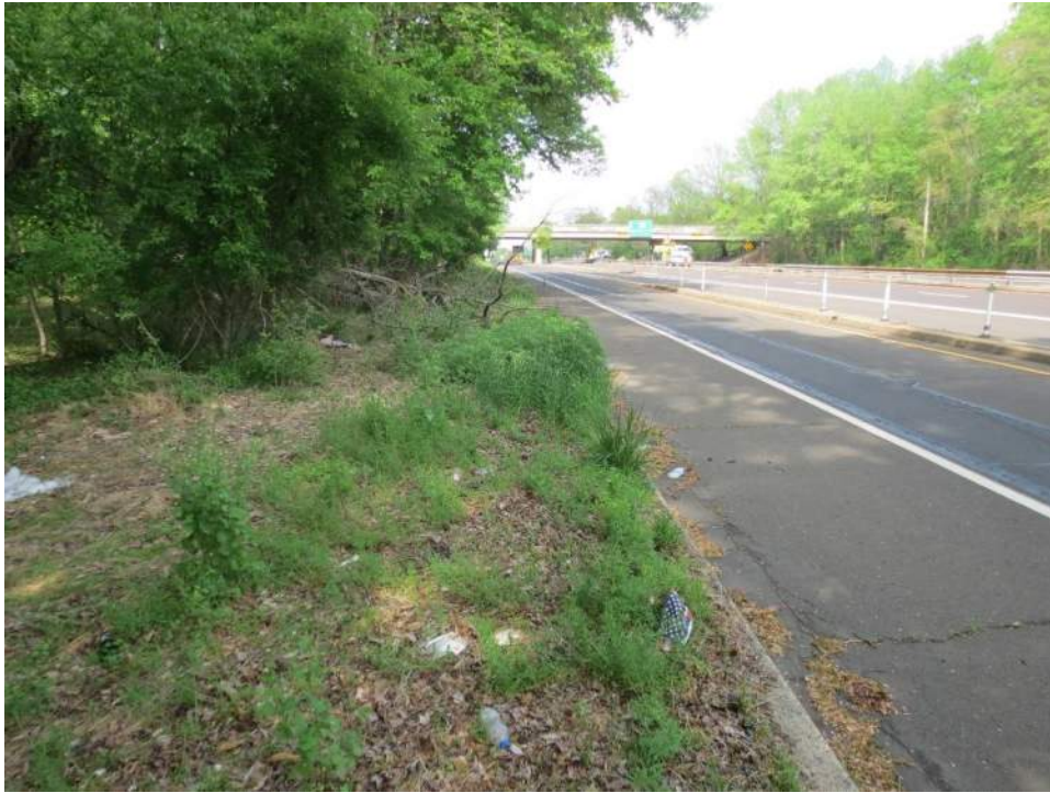
Photo 39: Looking northeast along the northern side of SR 0001, to the west of West Interchange Road. Photo taken May 4, 2021.
