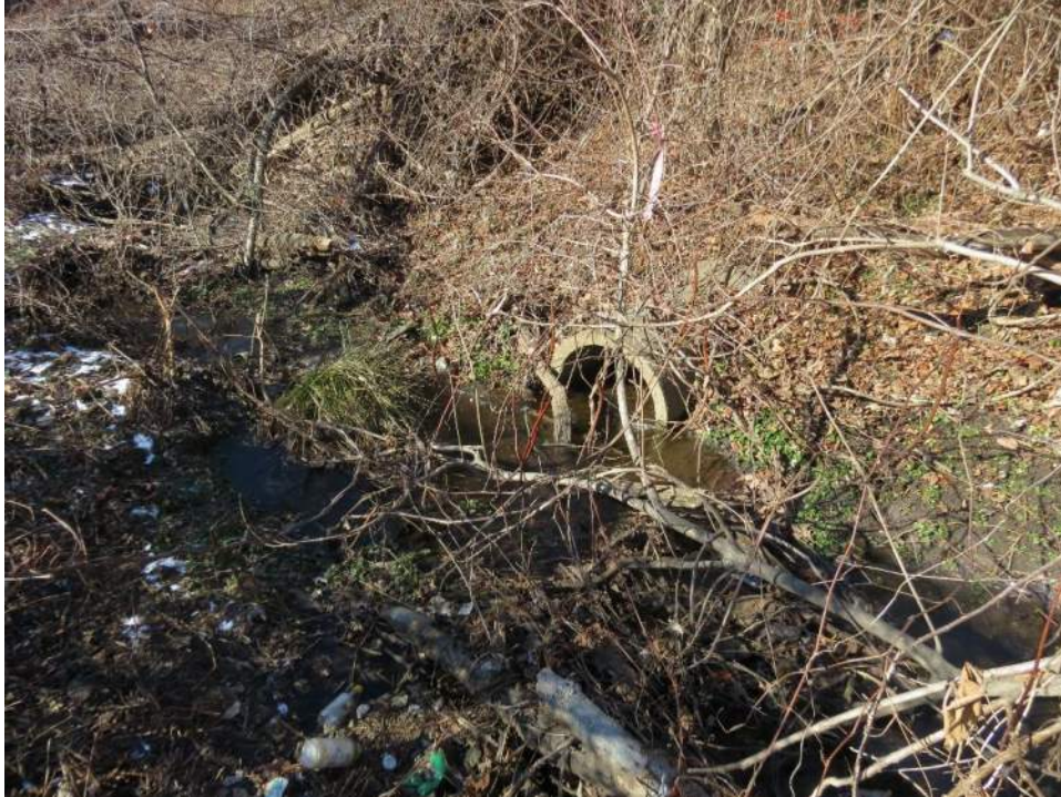
Photo 82: Looking northwest (upstream) along WUS-2, towards a stormwater pipe outfall that drains into the watercourse. Photo taken January 11, 2022.
