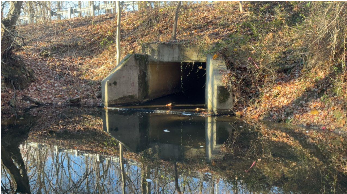
Photo 90: Facing northwest (upstream) along WUS-4 toward the culvert under West Highland Avenue in the central portion of the study area. Photo taken November 26, 2024.
