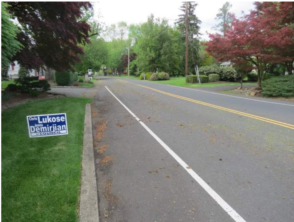
Photo 46: Looking north along SR 2047 (Hulmeville Avenue), to the north of SR 0001. Photo taken May 4, 2021.
