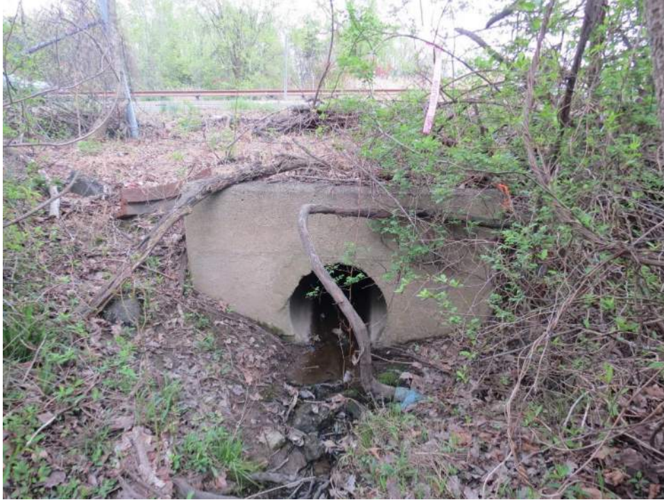
Photo 10: Looking southeast (downstream) along WUS-3 towards the pipe headwall on the northern side of SR 0001. Photo taken April 19, 2021.
