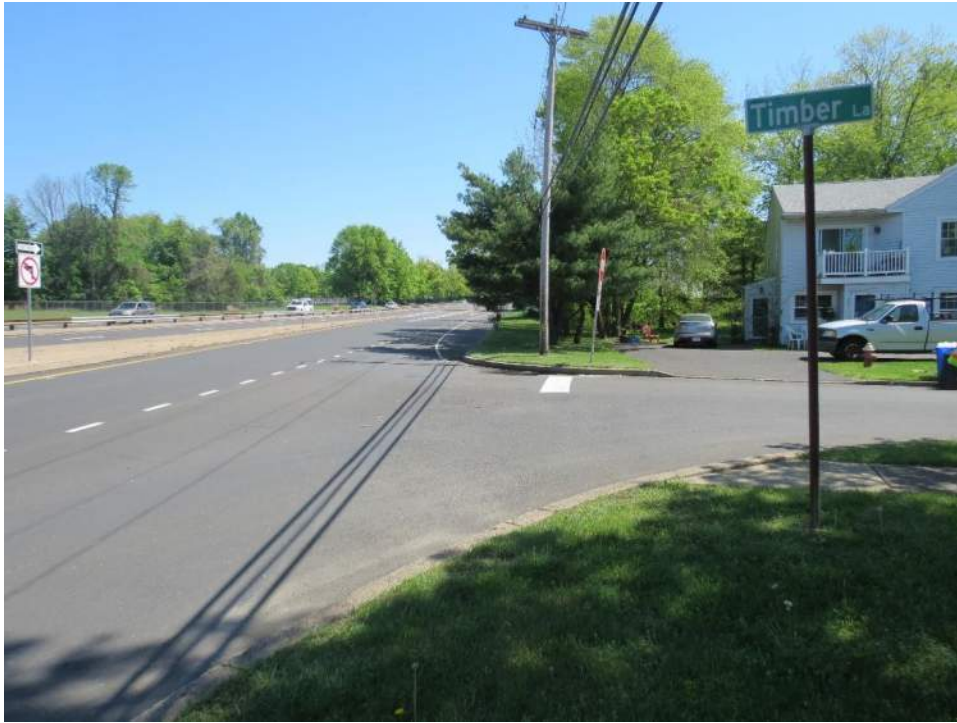
Photo 55: Looking northeast along the southern side of SR 0001, towards its intersection with T-824 (Timber Lane). Photo taken May 11, 2021.
