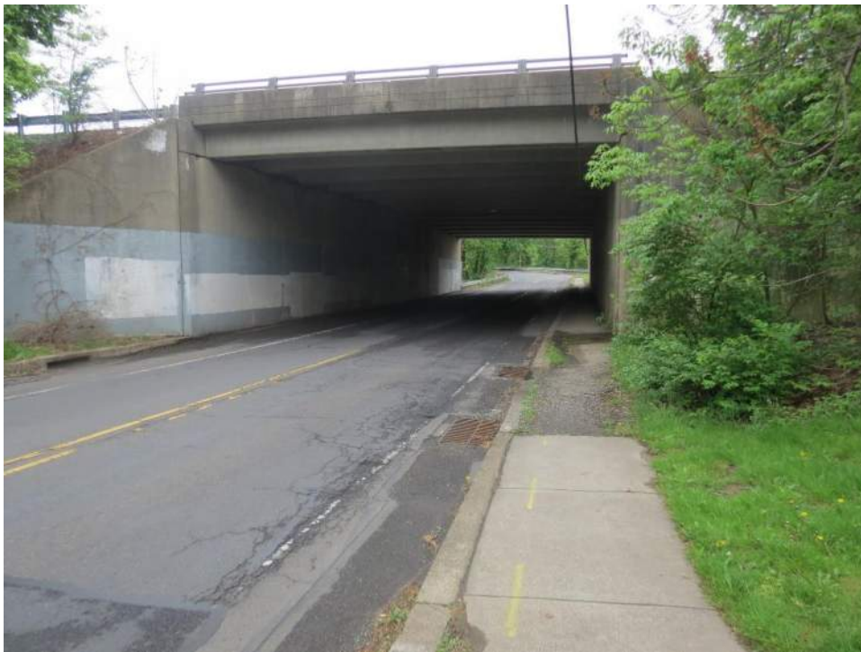
Photo 22: Looking southeast beneath the bridge carrying SR 0001 over SR 2008 (Highland Avenue), in the southwestern portion of the study area. Photo taken May 4, 2021.
