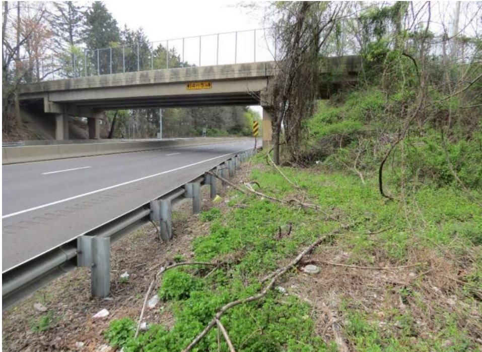
Photo 3: Looking southwest along SR 0001 southbound towards the Corn Crib Lane overpass, in the northeastern portion of the study area. Photo taken April 19, 2021.
