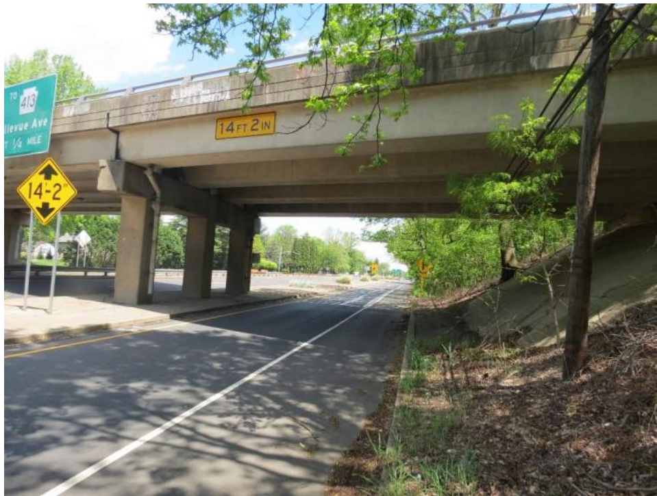
Photo 62: Looking northeast along the SR 0001 northbound frontage road, beneath the bridge carrying West Interchange Road over SR 0001. Photo taken May 11, 2021.
