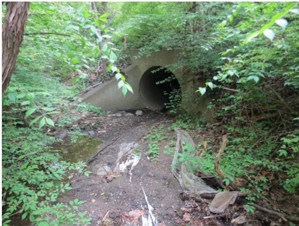
Photo 64: Looking southwest (downstream) along WUS-14, towards the culvert crossing beneath West Interchange Road. Photo taken May 11, 2021.
