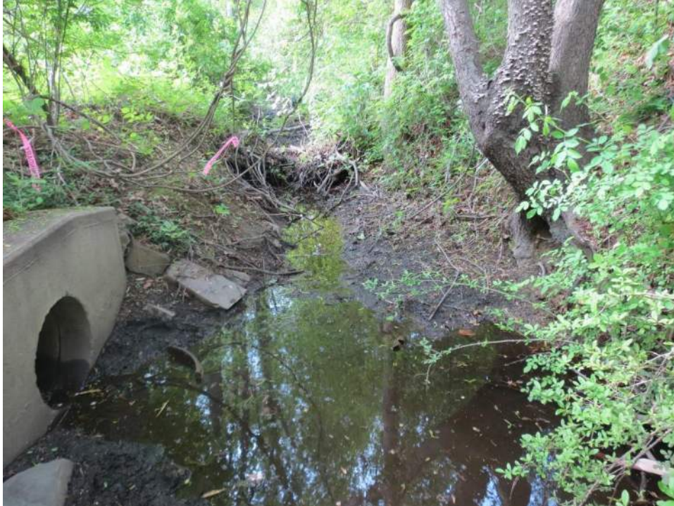
Photo 70: Looking northwest (upstream) along the southern end of WUS-2, to the south of SR 0001 and west of SR 0413 (Pine Street). Photo taken May 11, 2021.
