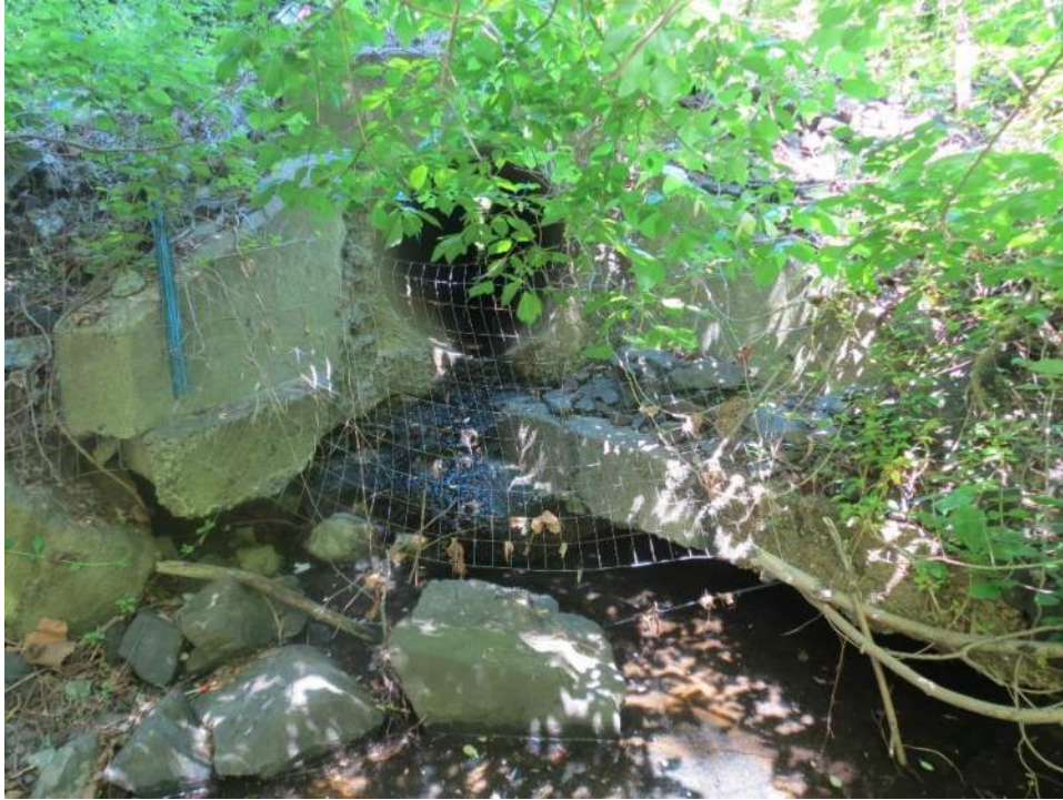
Photo 77: Looking northwest (upstream) along WUS-9 towards the culvert crossing beneath SR 0001. Photo taken May 19, 2021.
