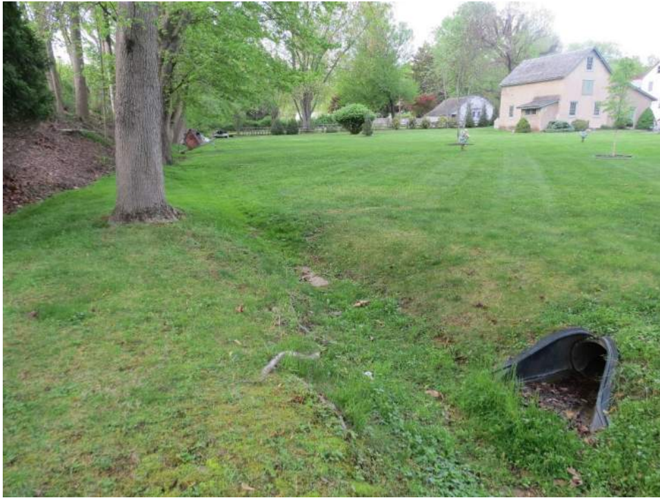
Photo 45: Looking north along grass drainage located just north of SR 0001 and east of West Interchange Road. Photo taken May 4, 2021.
