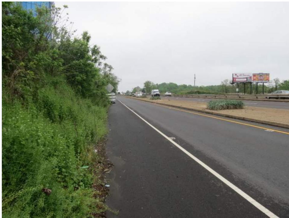
Photo 16: Looking northeast along the northern side of SR 0001, in the southwestern portion of the study area. Photo taken May 4, 2021.
