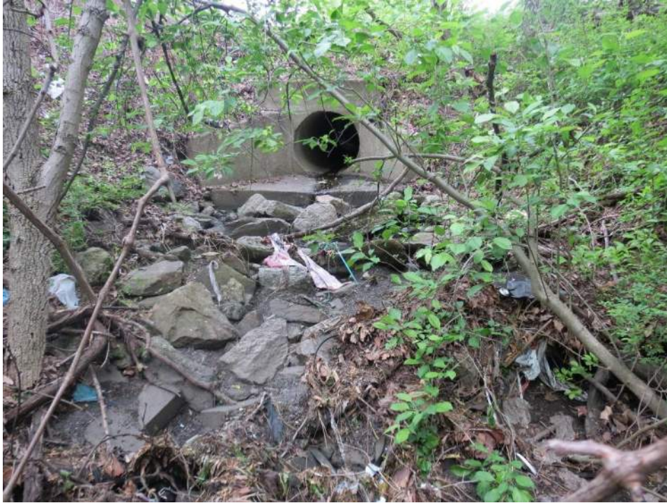
Photo 65: Looking north (upstream) along WUS-14, towards the culvert crossing beneath SR 0001. Photo taken May 11, 2021.
