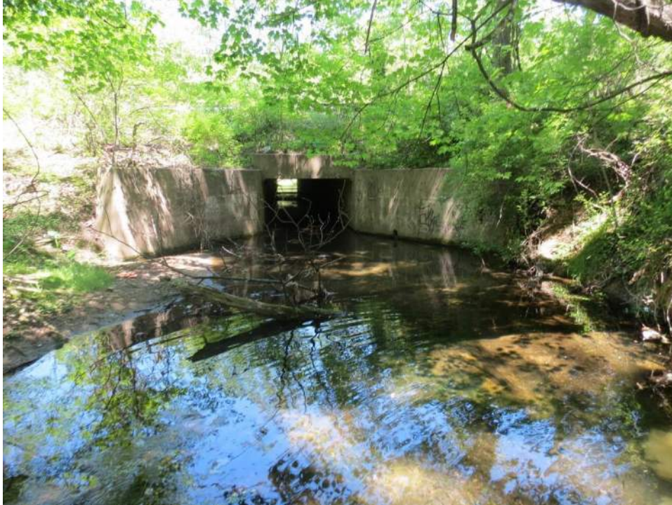
Photo 58: Looking north (upstream) along WUS-4, towards the culvert crossing beneath SR 0001. Photo taken May 11, 2021.
