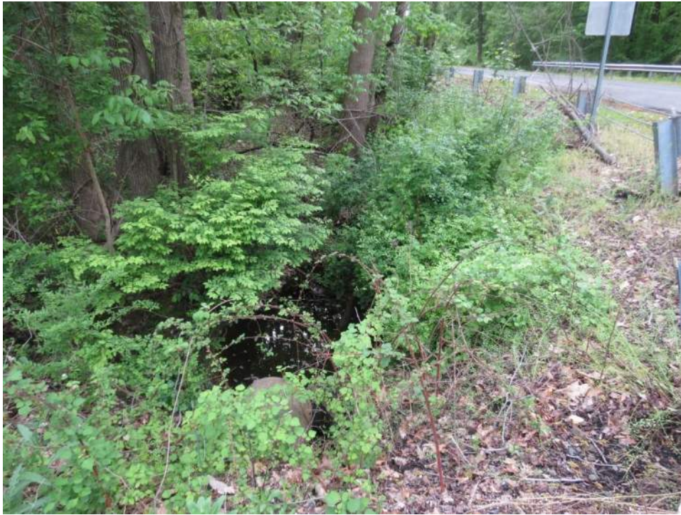
Photo 43: Looking west (downstream) along WUS-11, located at the northern end of West Interchange Road. Photo taken May 4, 2021.
