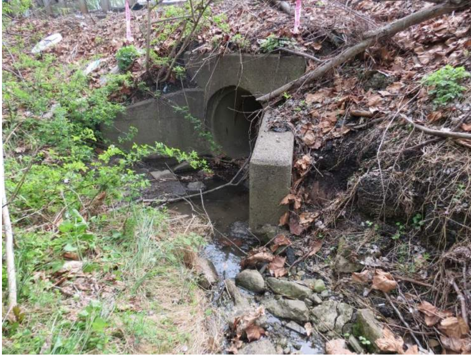
Photo 2: Looking east (downstream) along WUS-9 towards the headwall of the culvert crossing beneath SR 0001, in the northeastern portion of the study area. Photo taken April 19, 2021.
