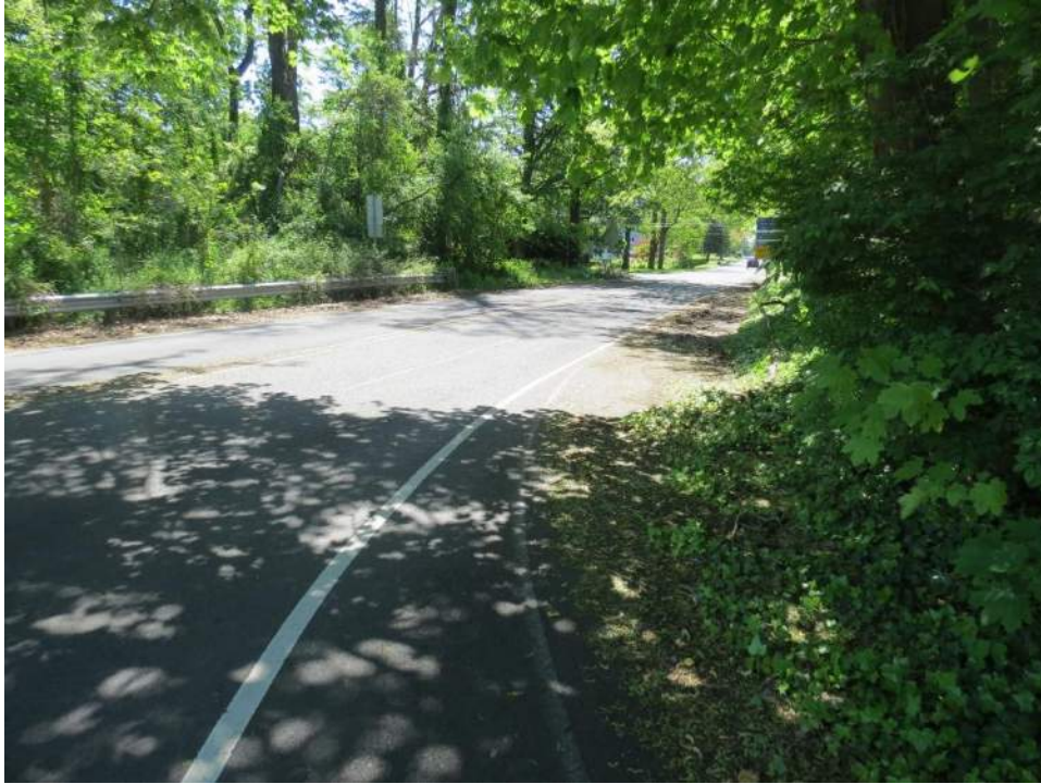
Photo 57: Looking southeast along SR 227 (Hulmeville Road), from its intersection with the southern side of SR 0001. Photo taken May 11, 2021.
