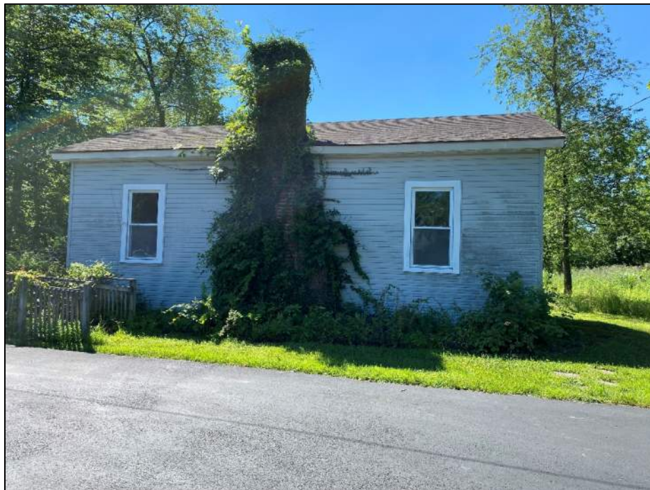
Photo 28: Structure on property adjacent to the parking lot in Photograph 27, facing south.
