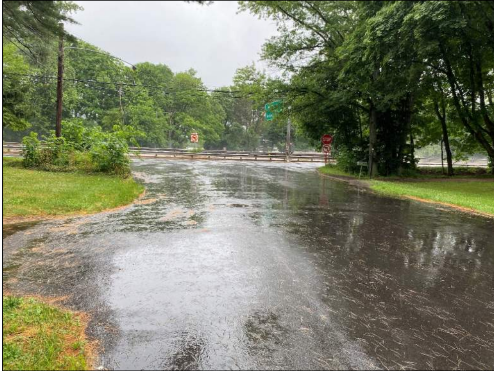
Photo 17: Looking at SR 0001 from Hill Avenue, facing northwest.
