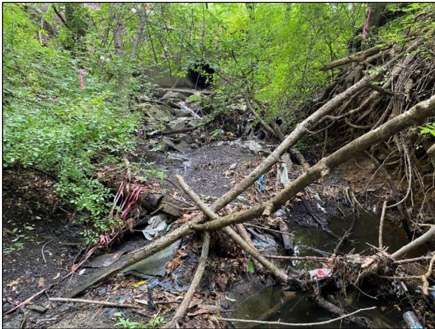
Photo 12: Culvert and stream running under SR 0001 parallel to West Interchange Road, facing northwest.
