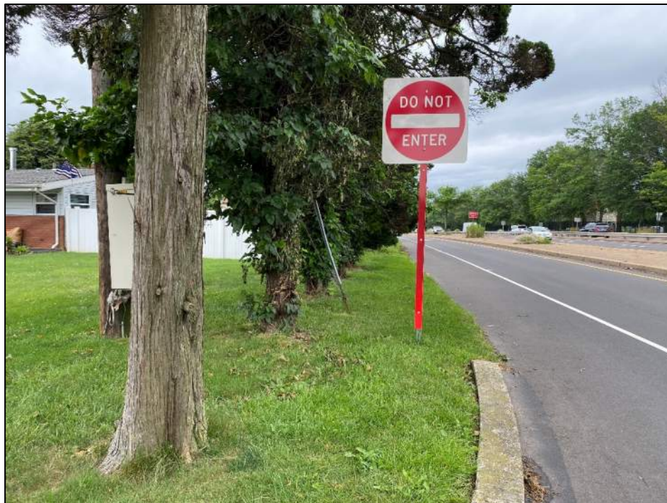
Photo 6: The service (frontage) road shoulder from Timber Lane, facing south.
