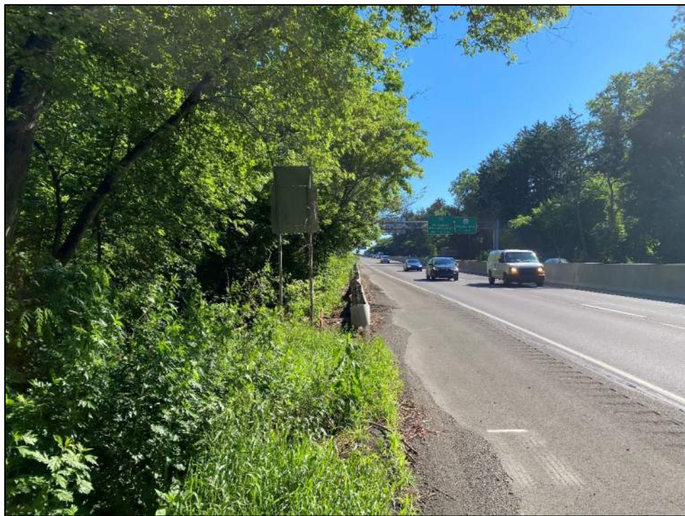
Photo 26: Southbound shoulder of SR 0001, facing northeast.
