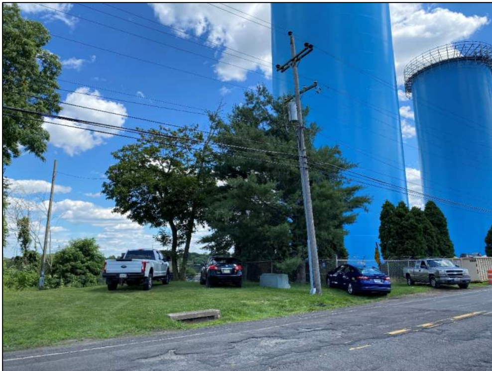
Photo 44: Bucks County Water and Sewer Authority (BCWSA) tanks, facing southeast. The BCWSA property is adjacent, but outside of the AOI.
