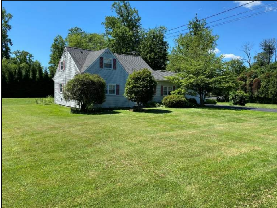
Photo 31: Property adjacent to the Langhorne Presbyterian Church located at 144 E Gillam Avenue, facing south.
