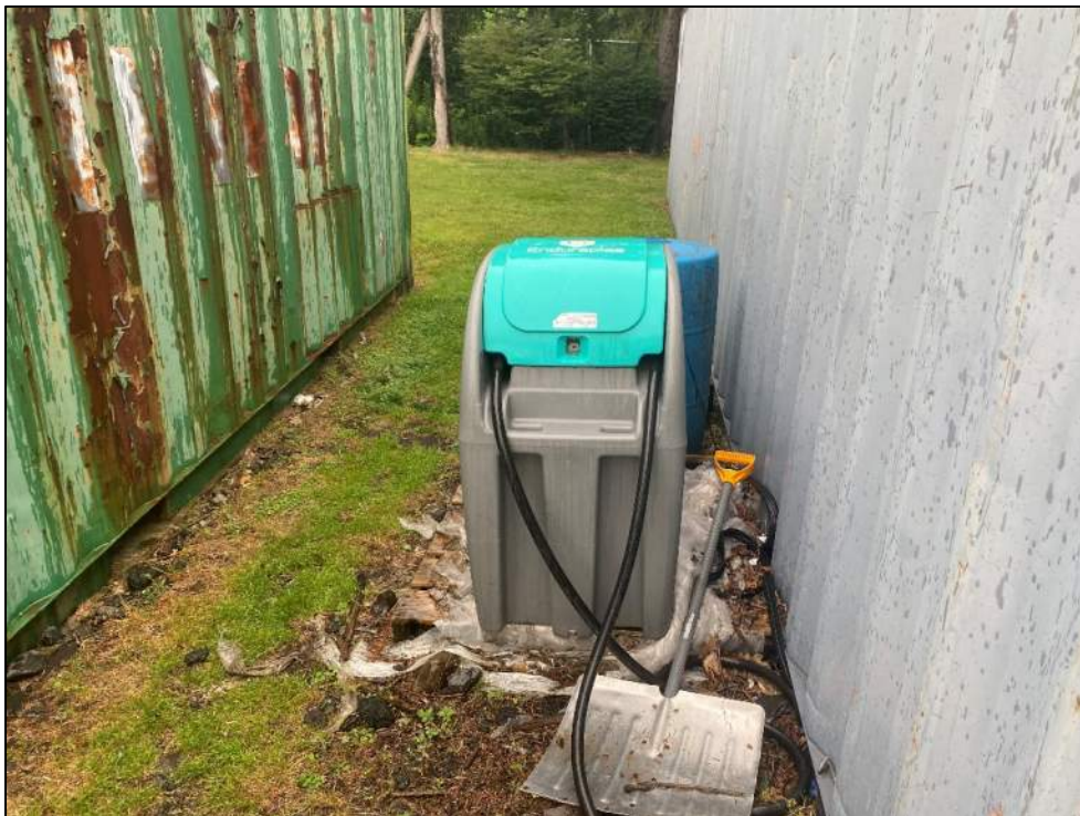
Photo 24: Plastic portable diesel fuel tank on the Woods School Property, facing northwest.
