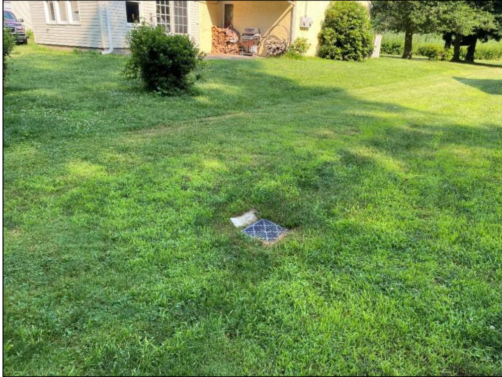
Photo 56: Stormwater drain in the backyard of the residence, facing northwest.
