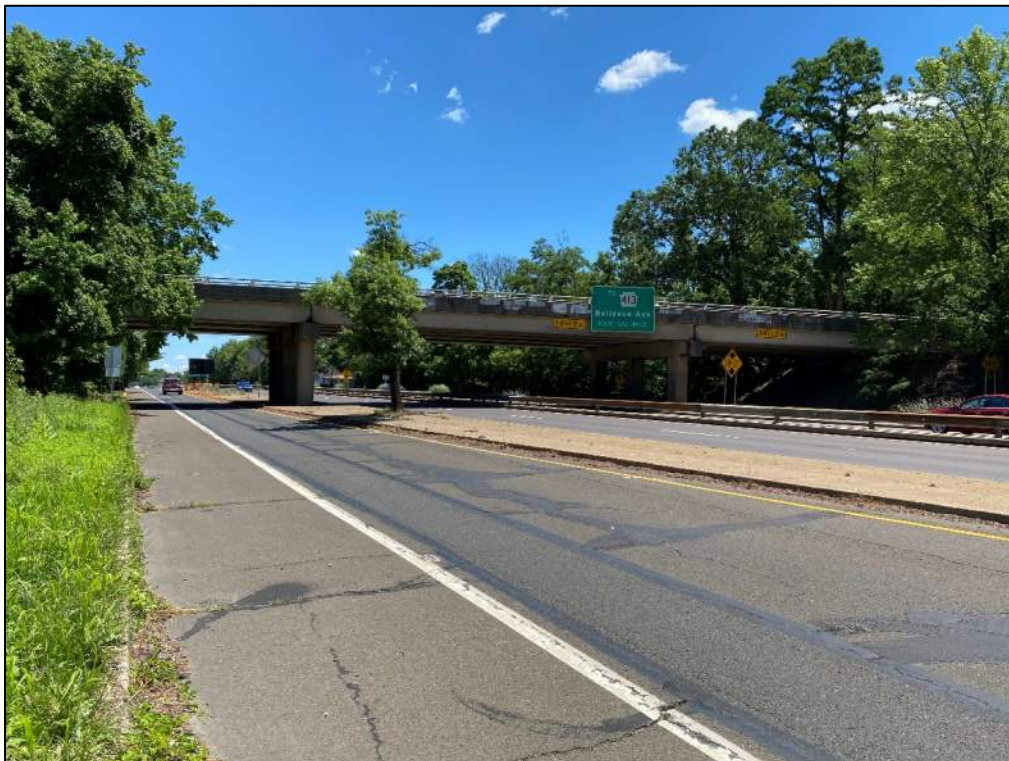
Photo 36: West Interchange Road overpass, facing east.
