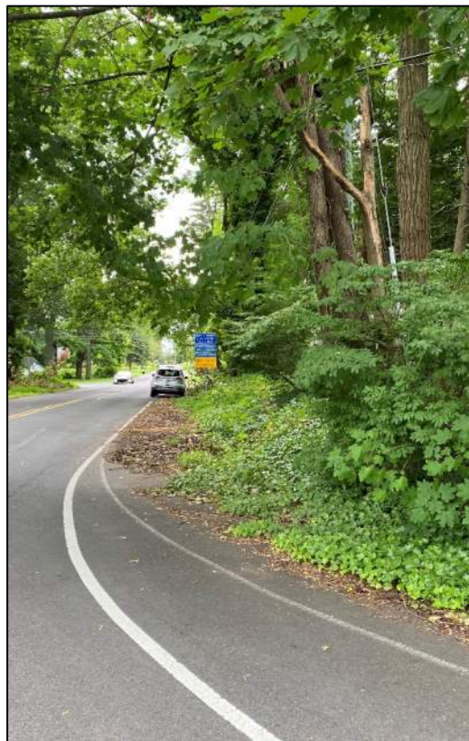
Photo 10: Hulmeville Road approach to the service (frontage) road, facing south.
