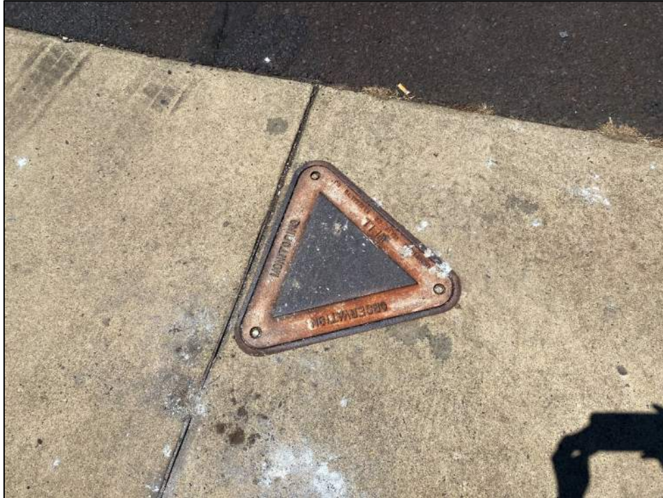
Photo 33: Monitoring well on Picernos Conoco gas station property. The wells were located outside of the AOI.
