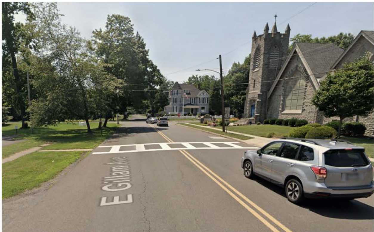
Figure 20A. Existing Condition of Gillam Avenue and Bellevue Avenue Intersection.
