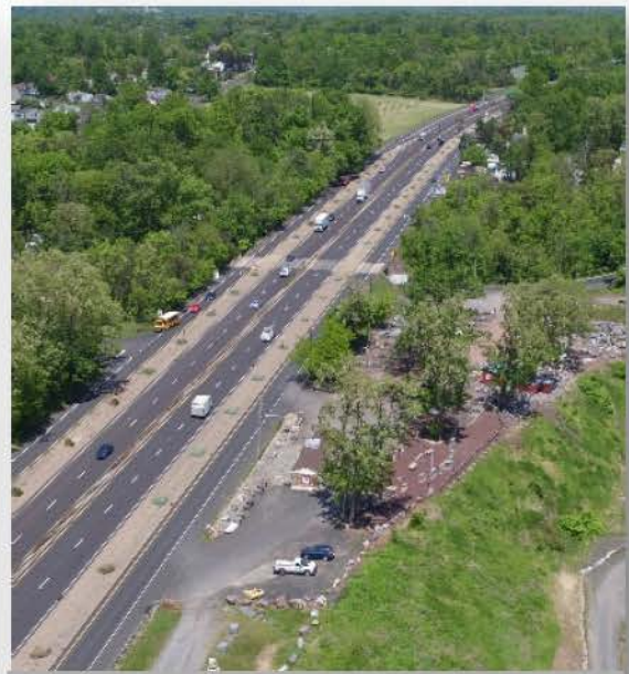
Photo 2. Aerial View Near Southern Project Limit (Looking North)
