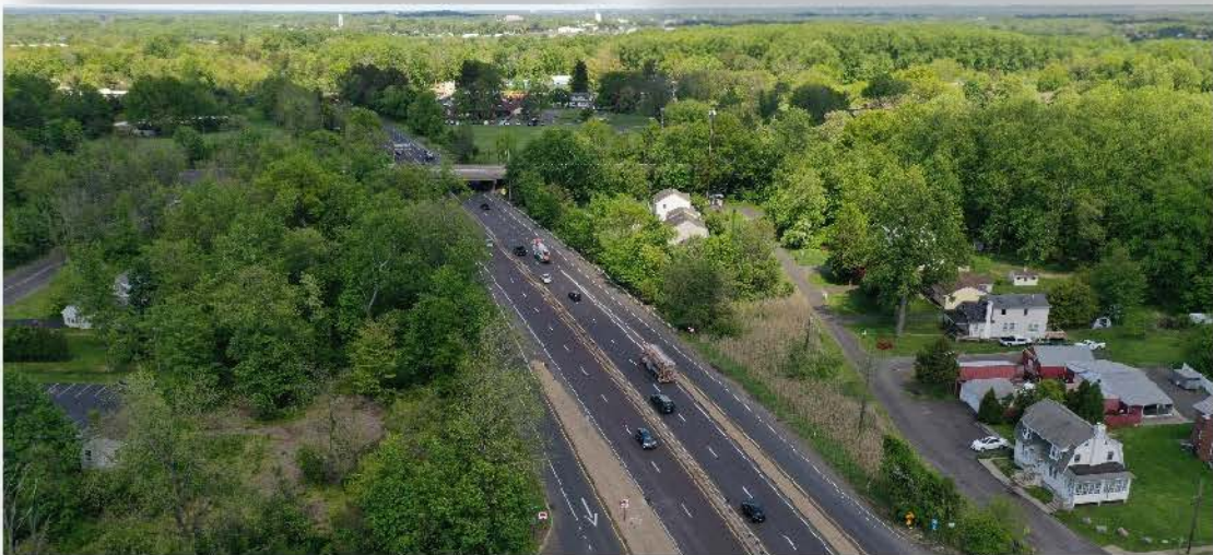
Photo 3. Aerial View of Gillam Avenue Intersection and SR 0413 Overpass (Looking East)
