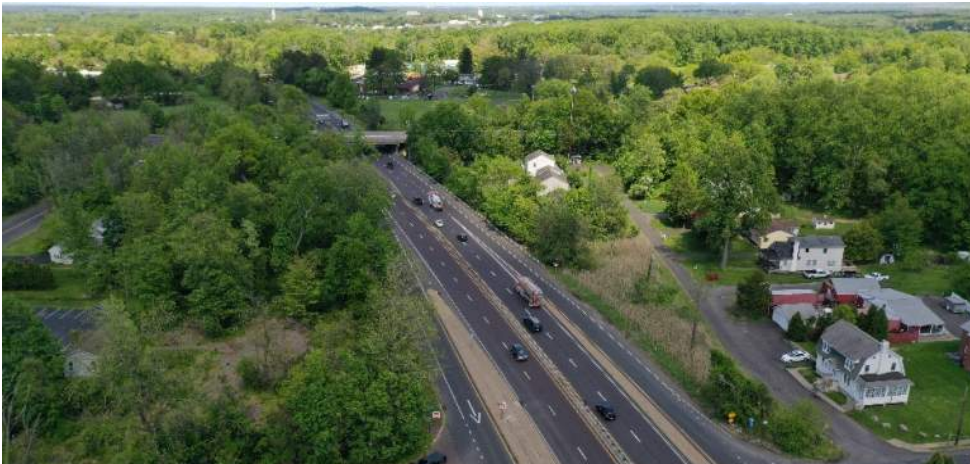
Aerial View of Hulmeville Avenue Intersection and PA 413 Overpass (Looking North)
