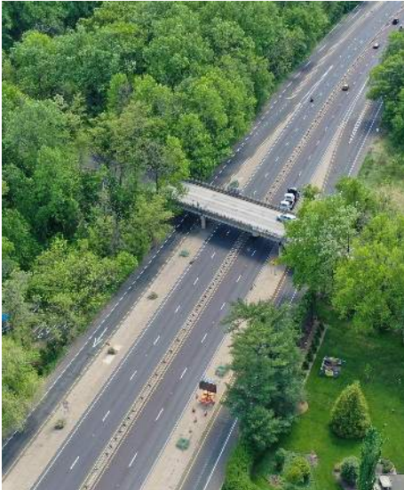
Aerial View of West Interchange Road Overpass (Looking South)
